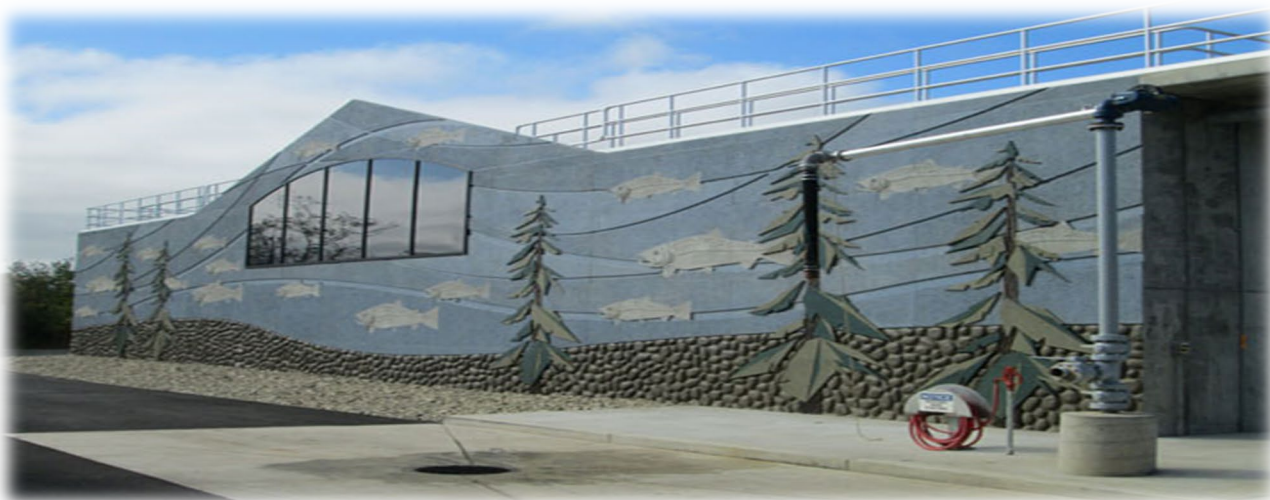
Photo Above: City of Coquille SBR with architectural windows and concrete artwork.
